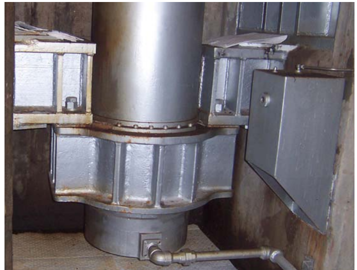
Lock No. 19 will be equipped with four 18-inch bore Eaton cylinders with custom machined flange mounting requirements.
